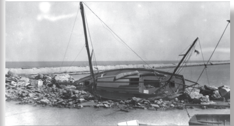
Storm Damage – Bad weather, particularly blows from the southeast, damaged many boats over the years. The Yacht Club would eventually build a pier system to prevent problems like this. RYC Photo, 1948
