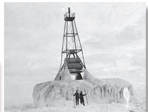
The first permanent Racine Reef Beacon. Tanks for the Pintsch gas used to fuel it can be seen at the bottom of the tower. Courtesy of the Racine Heritage Museum.
