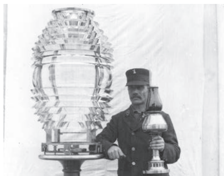
The 3rd order Fresnel lens from the Wind Point Light. The lens itself stands 4 feet 8 inches tall and its diameter is 39 1/2 inches. Courtesy of the Racine Heritage Museum.
