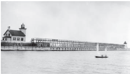
The Racine Harbor Lighthouse. Note the catwalk to the end of the pier. It gave the lighthouse keepers access to the light tower that can be seen at the end of the pier. Courtesy of the Racine Heritage Museum.
